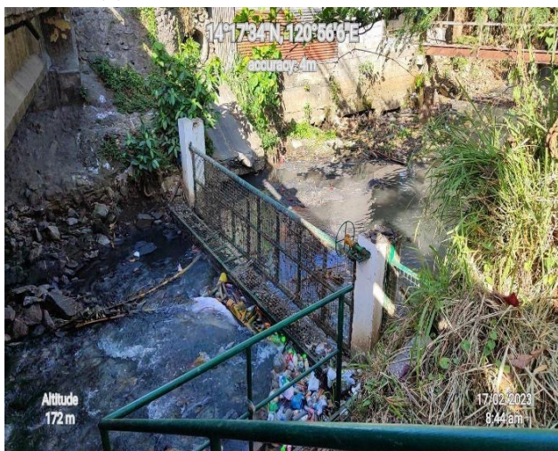
Figure 8-12. The (a - e) Designs and (f) Actual photo of the Collapsible-typed Trash Trap installed in Brgy. Langkaan I, Dasmariñas City, Cavite.
