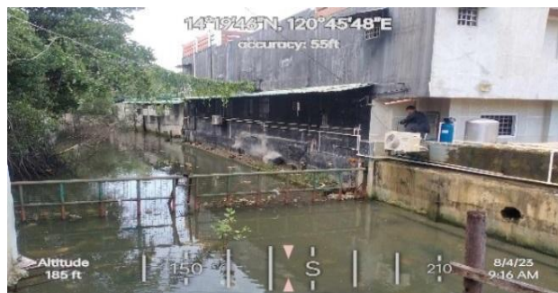
Figure 6 and 7. The (a) Design and (b) Actual photo of the Gate-typed Trash Trap installed in Brgy. Bucana Sasahan, Naic, Cavite.
